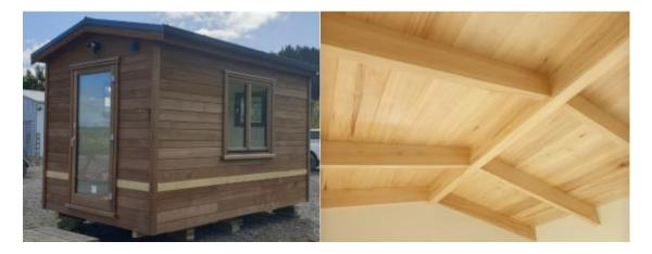
Photos: External view of cabin constructed from thermally treated 'Kawa' poplar; view of interior 'Kawa' poplar ceiling of the cabin.
